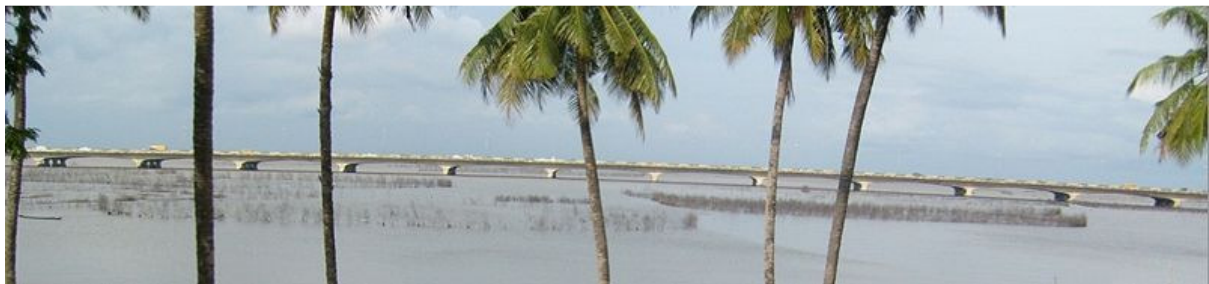
Third Mainland Bridge, Lagos
